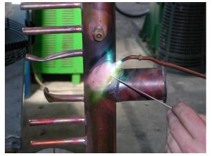
Following any damage causing the coil to break, having emptied the circuit the repair shall be carried out using braze-welding (for copper pipes), or TIG welding (for stainless steel pipes). Welding repairs must be carried out using the special alloys. For further information please contact your local Alfa LU-VE representative.
